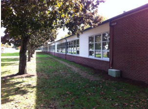
Exterior Elevation After
