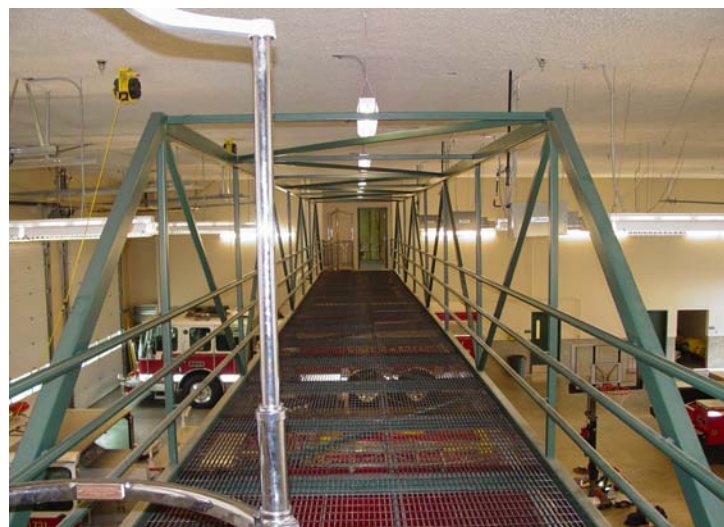
Looking across Bridge over Apparatus Bays
